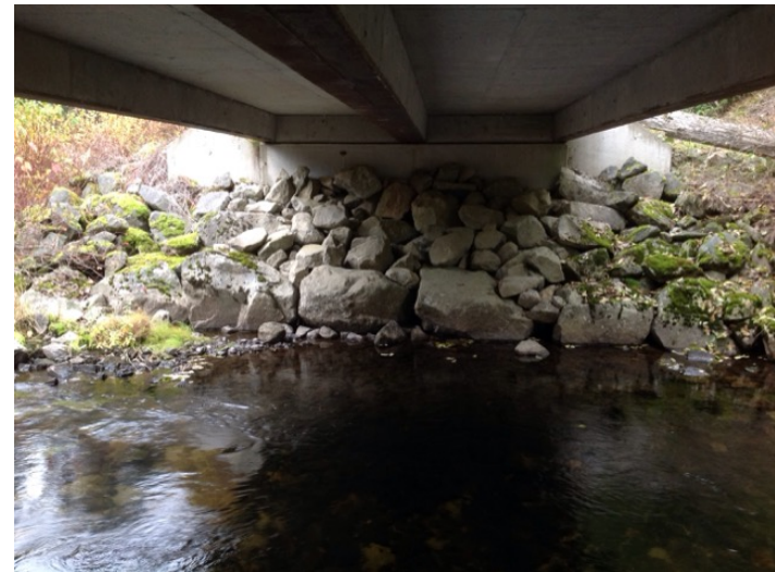
Left Bank Abutment when facing downstream
