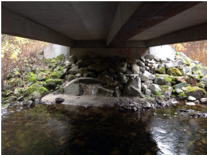
Right Bank Abutment when facing downstream
