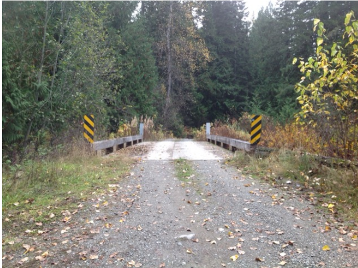
Approach from Left Bank when facing downstream
